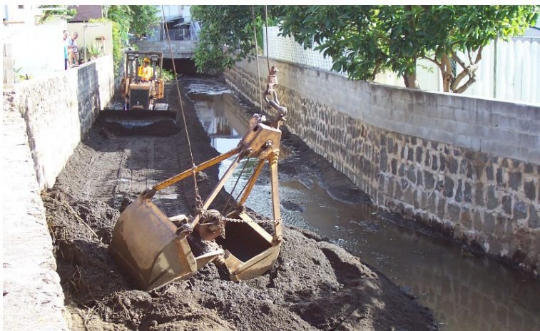
Workers cleaning debris from drainage channel.
