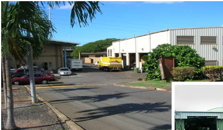
Pearl City Repair Facility
